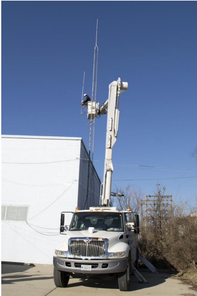
The old 224 MHz antenna is removed first KE0YI Photo
